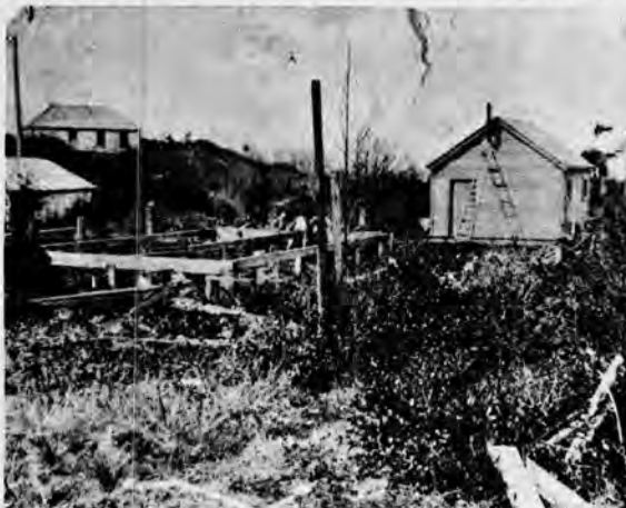
Foundation of O.I.C.'s house being constructed at Pachena Point (E. W. Kelk was O.I.C. at that time, 1923). The building up on the hill was the power house with 120 volts of storage batteries to operate the station equipment. Two Fairbanks-Morse horizontal gas engines drove the generators by belt for charging. No power was supplied to the houses. Kerosene lamps were used.
